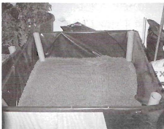
Bed fully constructed before soil is added. See the PVC pipes, the black plastic. Hydro-corals line the bottom and are then covered with felt and chicken wire.
